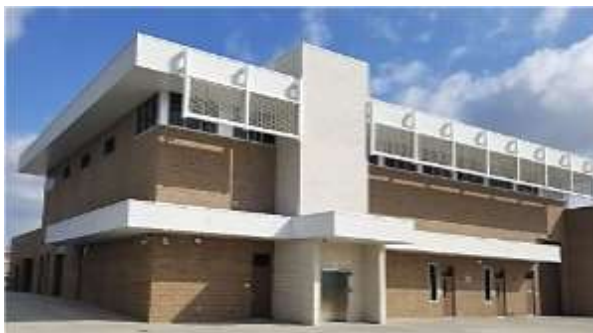
Figure 8. New Central Plant Building
