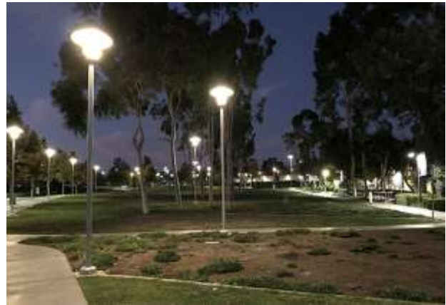
Figure 7. Exterior Lighting at Santiago Canyon College
