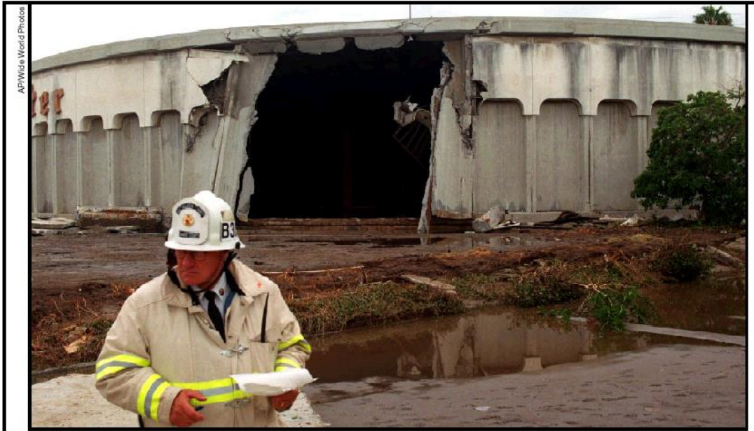
This 31-year-old storage tank ruptured in Westminster, California, sending a 6-foot wave of water through the city that damaged or destroyed about 50 buildings and over a dozen vehicles. Storage tanks should be replaced or periodically rehabilitated to preserve their structural integrity.
