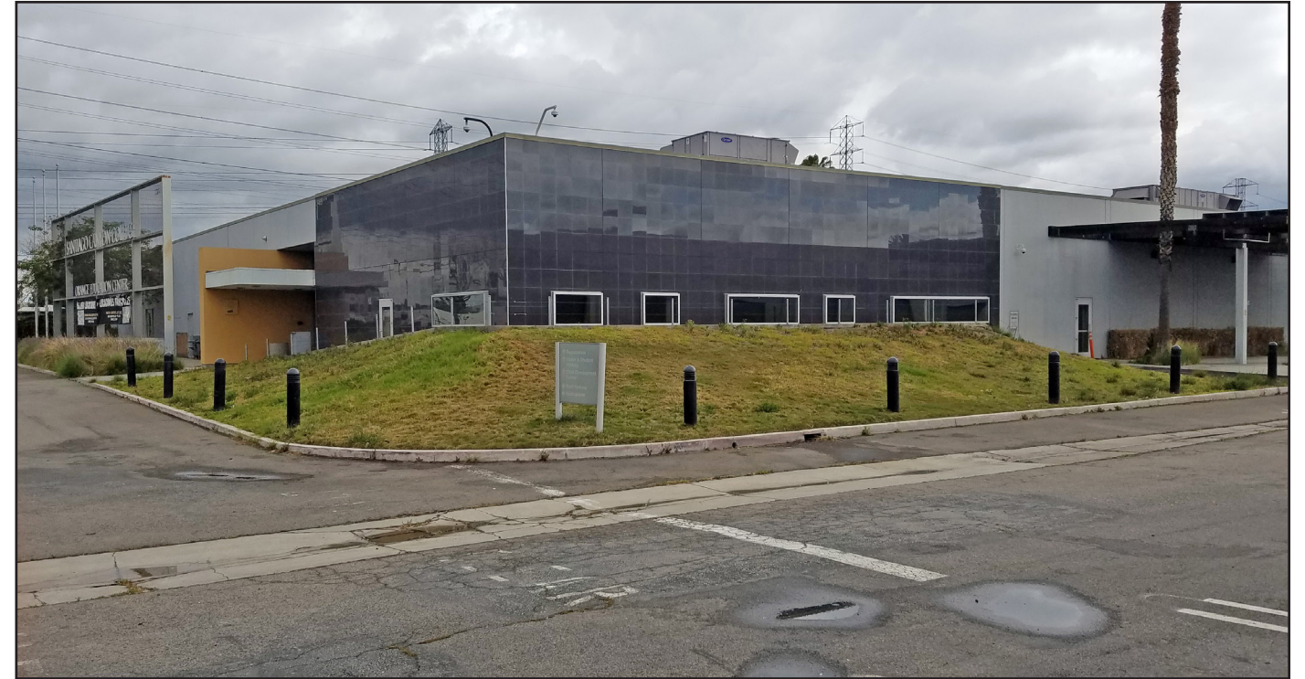
2. View of the southwest part of the OEC building looking northeast from the southwest part of the site.
