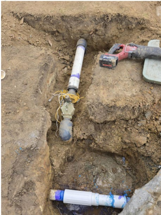
Valves Installed per SCC Request
