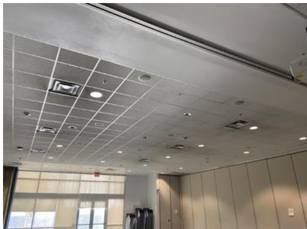
24 typical Ceiling mounted speakers in Staff Dining 116 & Cadet Dining 117 to be removed
