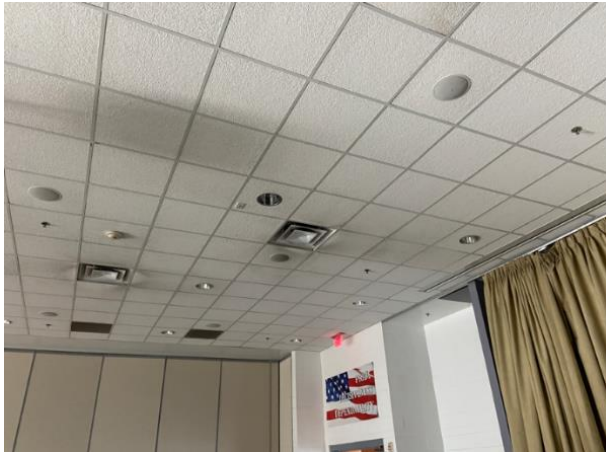
24 typical Ceiling mounted speakers in Staff Dining 116 & Cadet Dining 117 to be removed
