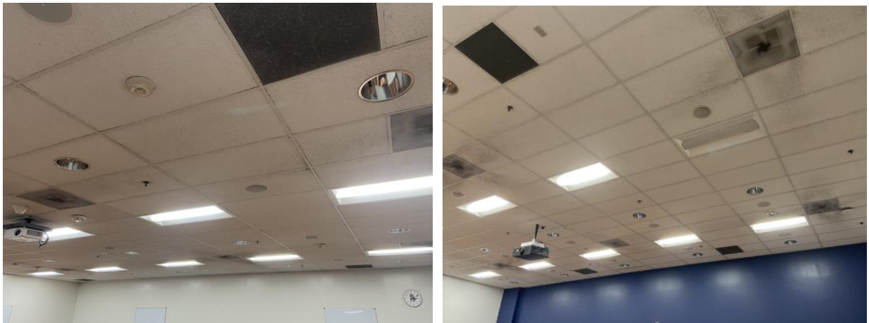
58 typical Ceiling mounted speakers & accessories in Classrooms 108, 111, 112 & 113 to be removed
