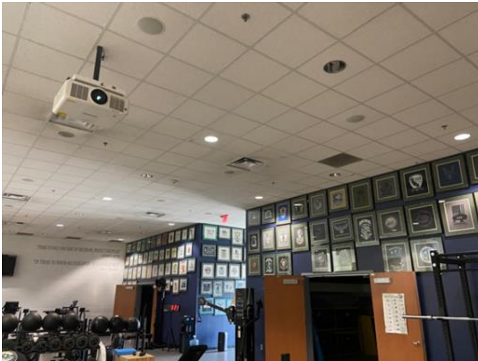
18 ceiling mounted speakers and accessories in Weight Room 119 to be removed
