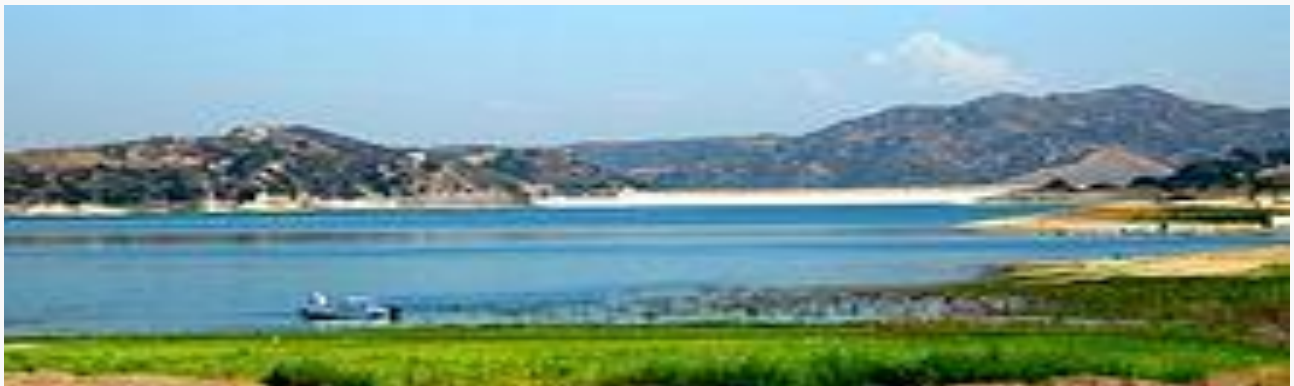
Santiago Dam, viewed from the eastern end of the lake
