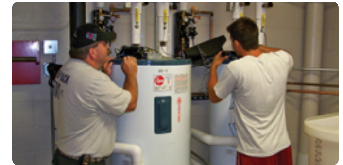
St. Clair County Community College students use data loggers to measure and analyze water temperatures as part of the new Siemens solar-powered hot water system in the college's Acheson Technology Center.
