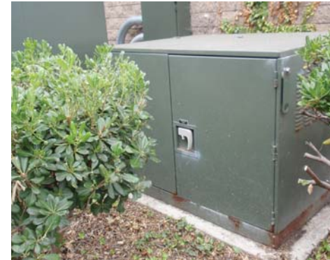
Typical Pad Mount 15KV Selector Switch
