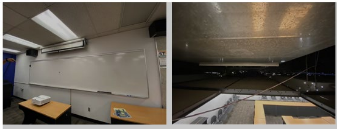
Existing Site & Ceiling Space Conditions in Room A 209
