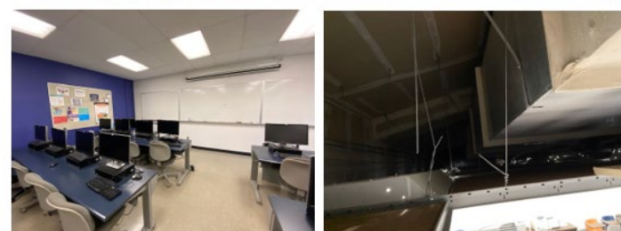
Existing Site & Ceiling Space Conditions in Room B 207
